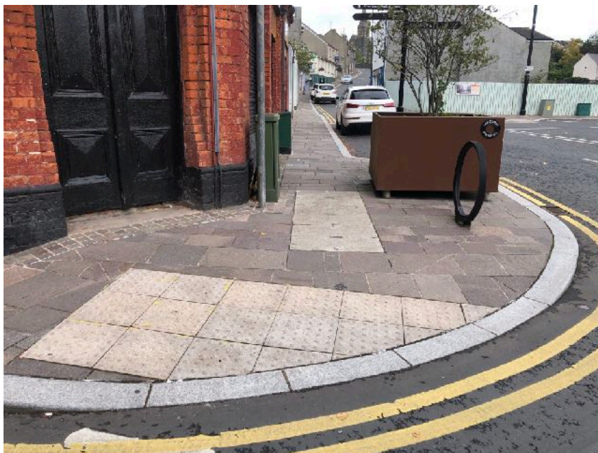
Image above shows the large planters and cycle stand used on the already narrow footways around Market Square, Dromore.
