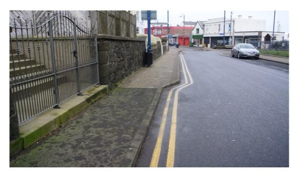
There is an uncontrolled crossing across Eglington Street just before the junction with Causeway Street and Main Street. The tactile paving does not contrast sufficiently with the surrounding paving.
