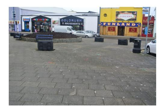
There is another uncontrolled crossing at this point providing access to and from the car park. The tactile paving does not contrast sufficiently with the surrounding paving.
