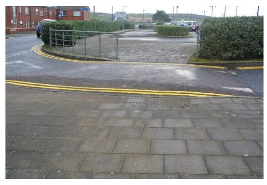
There is a controlled crossing providing access to the eastern footway on Dunluce Avenue. The tactile paving has been installed incorrectly on this crossing and the contrast with the surrounding paving could be improved.
