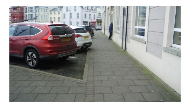
Uncontrolled crossings have been provided across both Mark Street and Causeway View to enable pedestrian access to the remainder of Main Street. The tactile paving does not contrast sufficiently with the surrounding paving.
