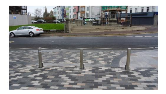
A further controlled crossing is provided from the traffic island to the eastern side of Eglington Street opposite to the Spar. Tactile paving has been installed incorrectly on this crossing.
