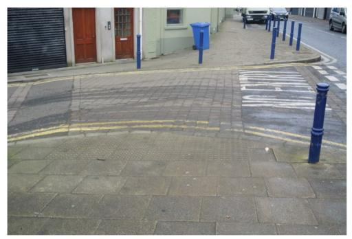
At the junction with Eglinton Street there is a section of dropped kerb providing access to the traffic island between Kerr Street and Eglinton Street. There is no tactile paving provided at this uncontrolled crossing.
