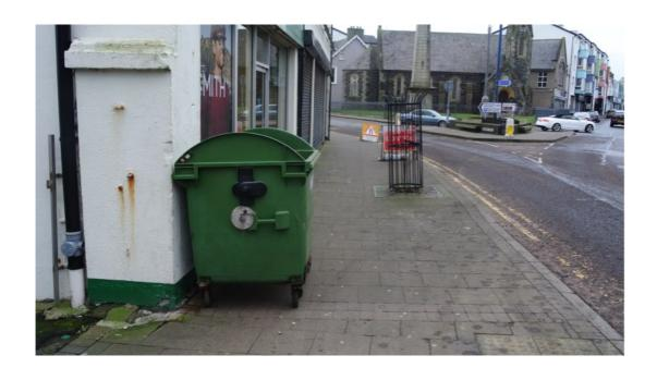
An uncontrolled crossing is provided across the junction with Manse Avenue on the western side of Main Street. Lack of contrast and tactile paving is again an issue as is the location of litter bins as is a cross fall on the footway.
