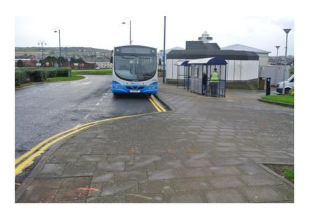
One of the main car parks for the town is located directly opposite the bus stops. An uncontrolled crossing is provided from the car park to the footway on the western side of Dunluce Avenue. Tactile paving has been laid incorrectly and fails to provide an adequate contrast with the surrounding paving.
