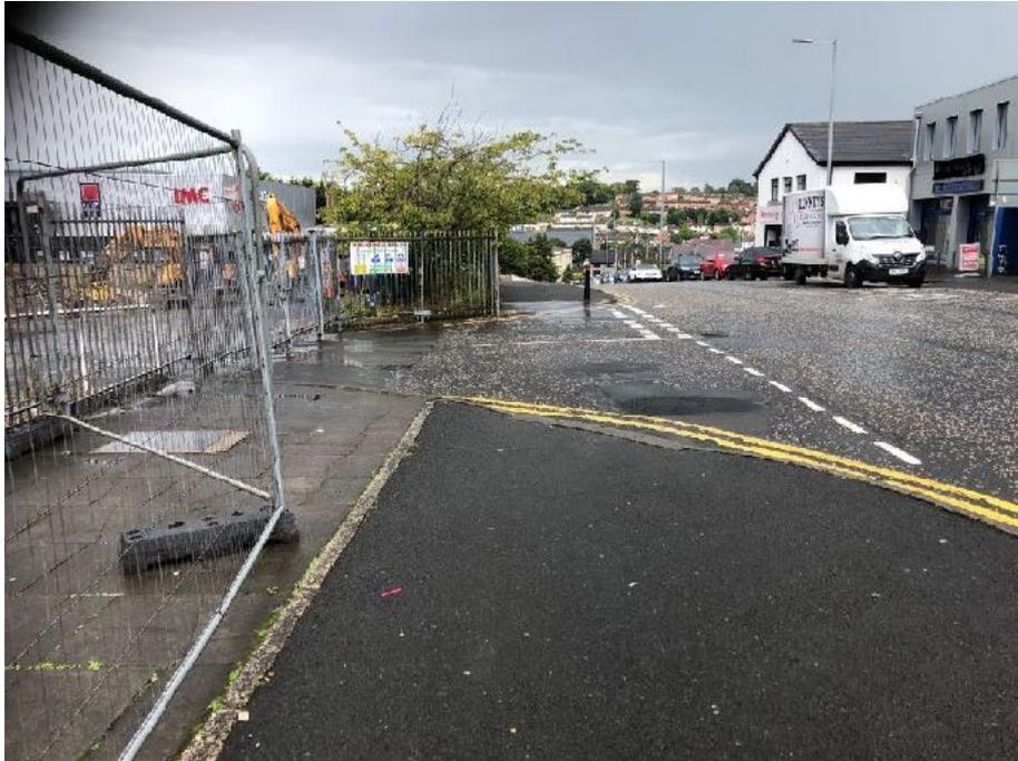
There is a dropped kerb without tactile paving on the western footway level with the entrance to the car park on eastern footway. A parking bay on the eastern carriageway obstructs access to the dropped kerb on the eastern footway.
