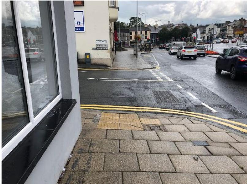
The footways on Burnview Terrace linking to the car park are narrow and in poor condition. Shop displays create obstructions on the northern side.
