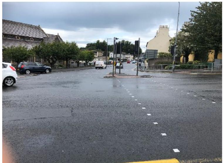
There is an uncontrolled crossing at the junction with Burnview Terrace. The tactile paving is laid correctly but damaged in places. There are sections of dropped kerb without tactile paving presenting a potential hazard for people with visual impairment. Contrast between the tactile paving and surrounding pavement could be improved.
