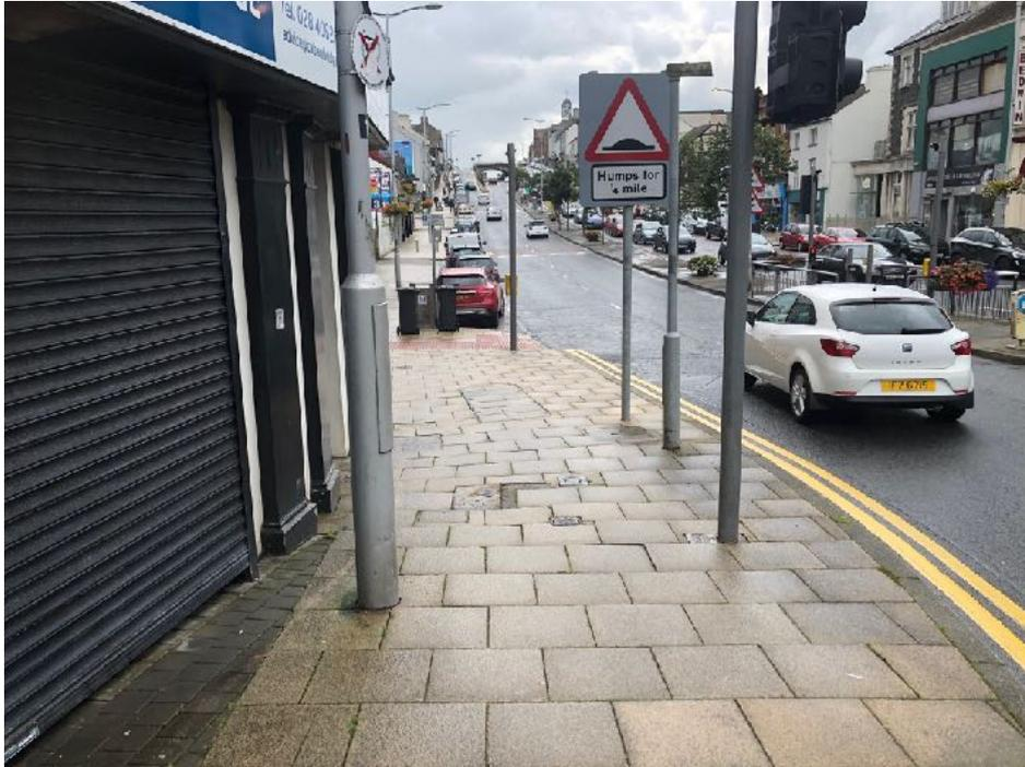
There is a controlled crossing across Bridge Street close to the junction with Church Square. The crossing is staggered with a traffic island at its mid point. Pedestrian railings have been provided on the island. Tactile paving and control boxes have been installed correctly.
