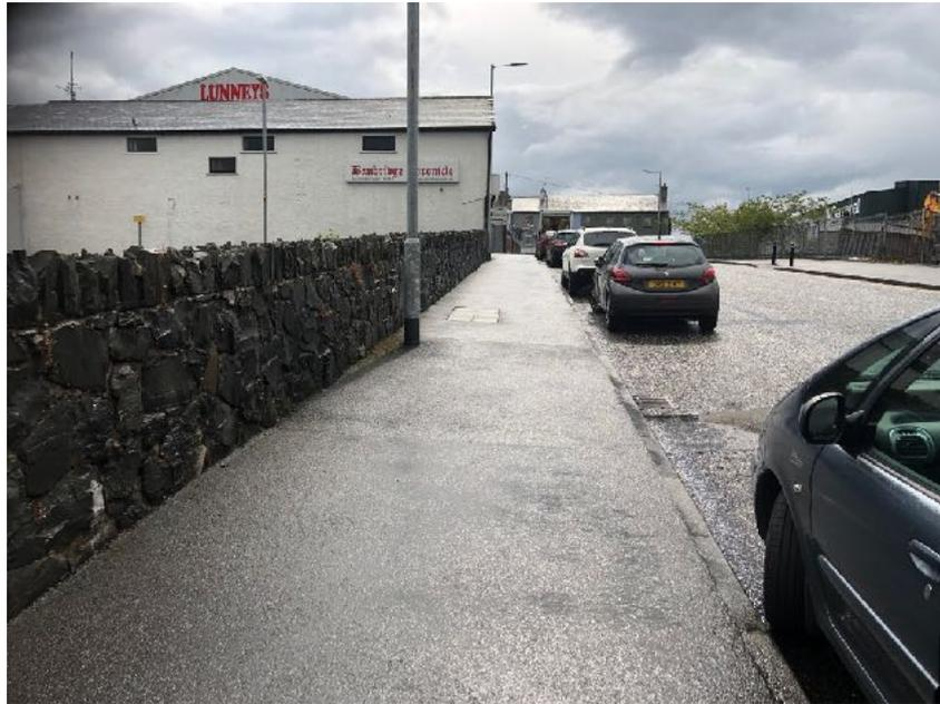
Ramped pedestrian access to the car park is provided close to this point. A handrail has been provided on one side but the surfacing and gradient of the ramp should be improved.
