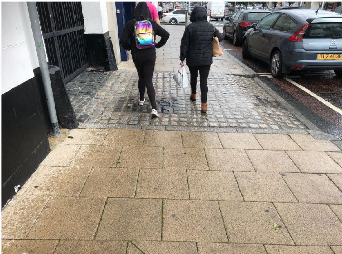
There is an indented uncontrolled crossing across the junction with Linenhall Street. Although the tactile paving has been installed correctly it does not contrast sufficiently with surrounding pavement.
