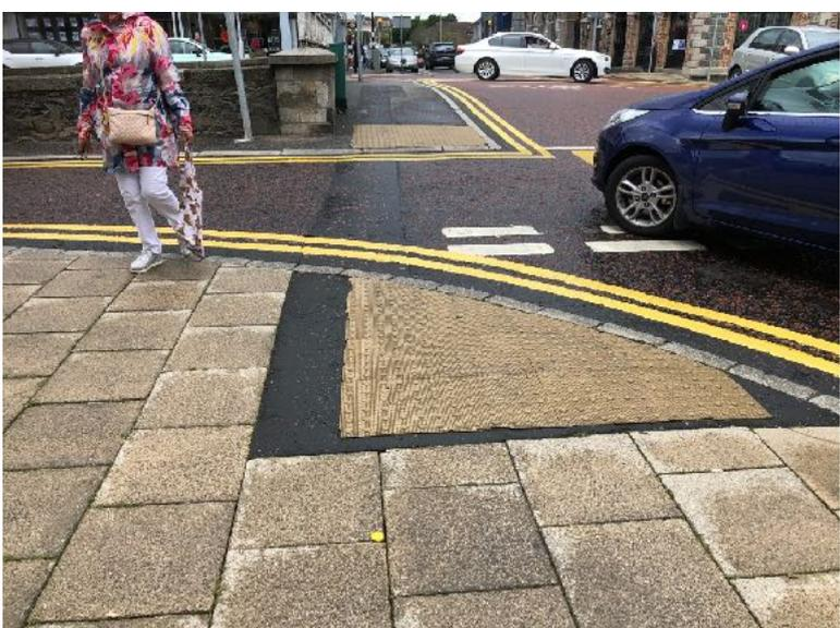
Uncontrolled crossings have been provided across Scarva Street and Rathfriland Street. Tactile paving layout does not meet standards. The tactile paving does not sufficiently contrast with surrounding pavements in places. The associated bollards do not include a strong visibility strip.
