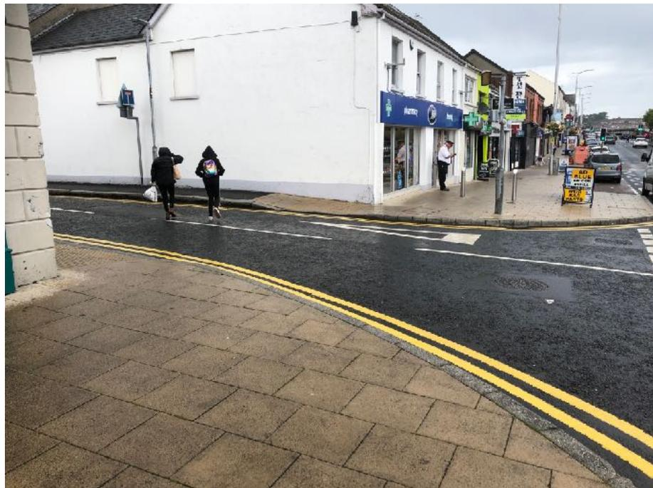
The footways on Linenhall Street are narrow, with street furniture on both sides further reducing available width, and in poor condition. There is no step free access along the length the southern footway.
