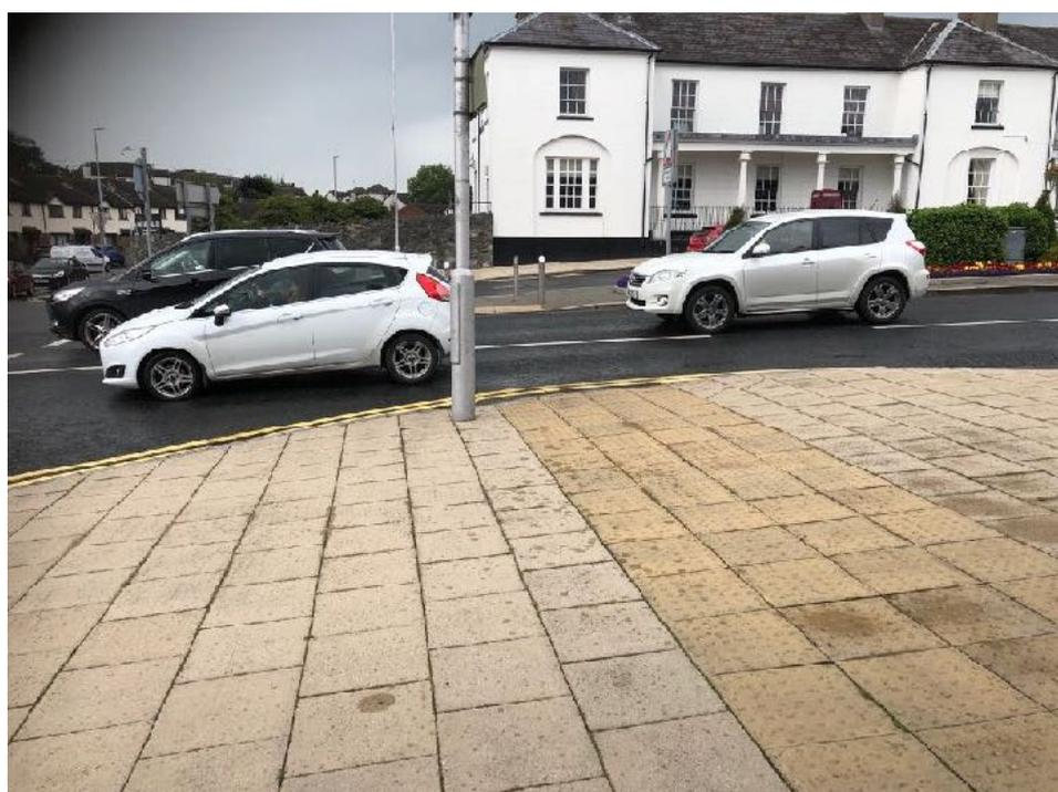
There is a series of uncontrolled crossings including a central refuge across Kenlis Street, Newry Road and Commercial Road close to the roundabout. The tactile paving is not be laid in accordance with standards. Even it was the heavy traffic levels at the roundabout means many disabled people cannot cross without assistance.
