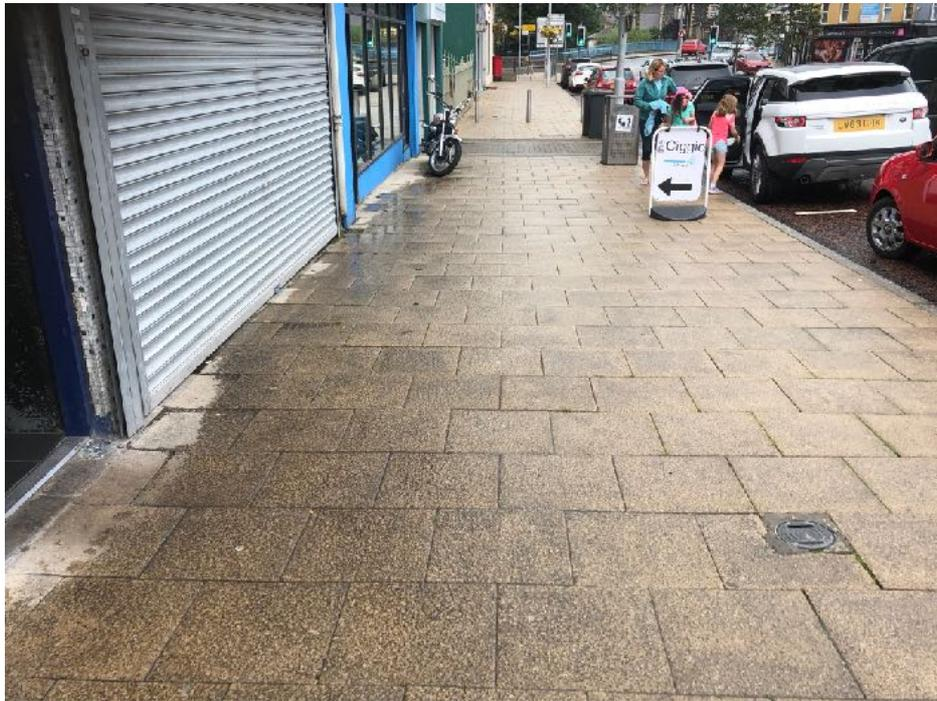
Two linkages either side of the Imperial Public House provide access to the Downshire Place off street car park. The area is dated with poor surfaces and in need of improvement. One access point to the car park is stepped although a step free alternative is available via a dropped kerb without tactile paving provided.
