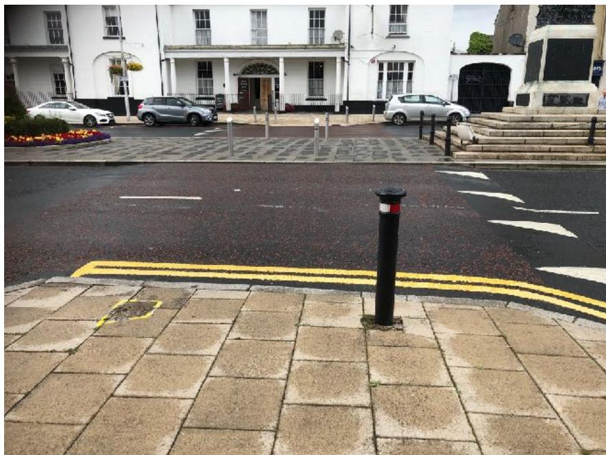
There is an uncontrolled crossing close to the roundabout at the end of Newry Street. The paving has not been laid to standard as it extends to the building line. The tactile paving does not sufficiently contrast with the surrounding pavement.
