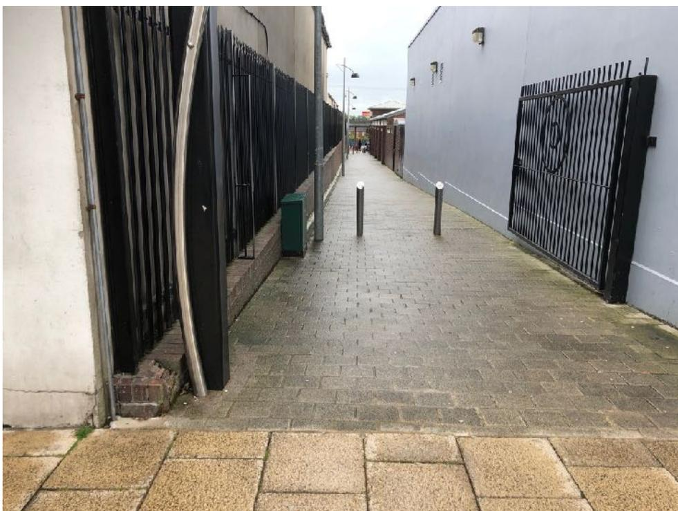
There is an indented uncontrolled crossing across Old Kenlis Street. Appropriate tactile paving has been provided. However this does not contrast sufficiently with the surrounding pavement.
