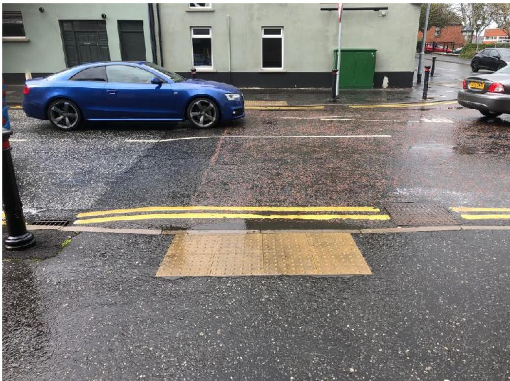
On the northern footway there is no uncontrolled crossing across Downshire Place. No dropped kerbs or tactile paving has been provided at this junction.
