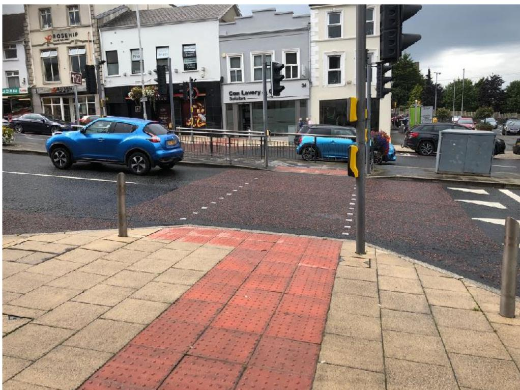
The gradient of the footway increases significantly after this point, approaching the historic bridge. A vehicle entrance with some kerb show and clutter from shops create potential hazards and the position of street lighting columns impact on clear footway width.
