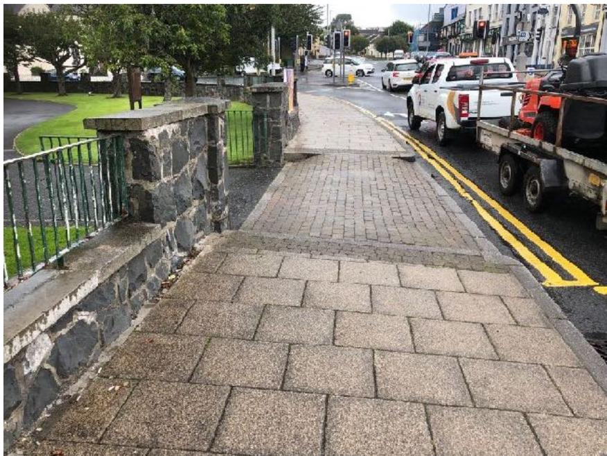
There are a series of complex controlled pedestrian crossings across Church Street at its junctions with Church Square and Dromore Street. Although tactile paving and control boxes have been installed correctly, the angular design of crossings at the junction means some disabled people will find using it very difficult or impossible without assistance.
