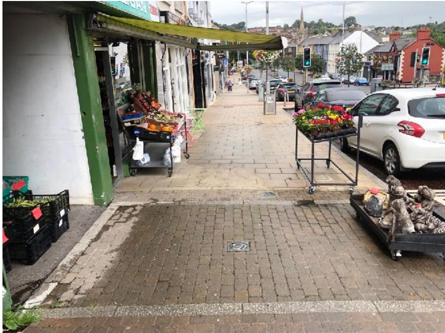
There is an uncontrolled across Bridge Street at the junction with Victoria Street. Although tactile paving has been installed correctly, it does not contrast sufficiently with surrounding paving.
