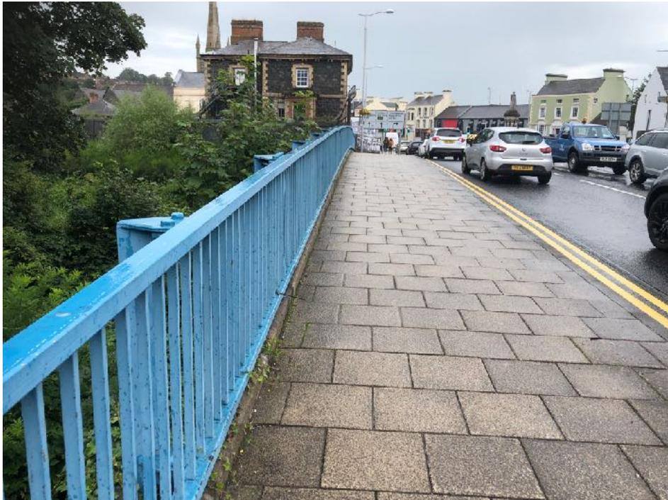
The western footway is significantly narrowed by building works after the bridge. This is no ideal on what is a very heavily trafficked area. Traffic signage poles create additional hazards.
