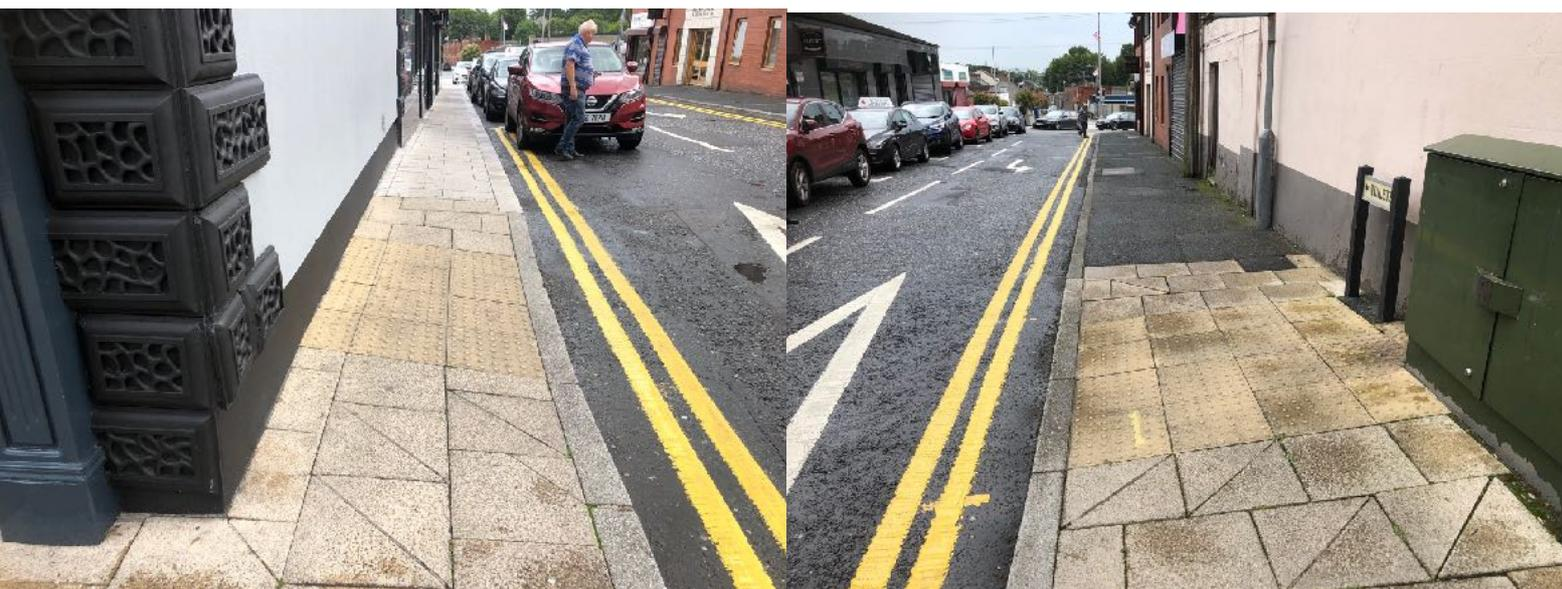
On Newry Street the carriageway is raised flush with the footway close to the Cenotaph, giving the impression this is an uncontrolled crossing. However no tactile paving has been provided making this a potentially hazardous place for people with a visual impairment. The visibility strip on bollards needs to provide a stronger contrast.
