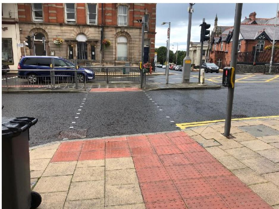
Although the eastern footway is broad the lack of consistency in the location of street furniture including bollards and lighting columns as well as vehicle entrances with kerb shows close to the carriageway create potential hazards for people with visual impairment.
