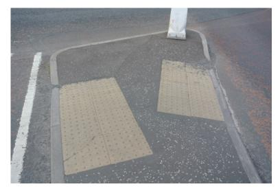
There is a good example of a controlled crossing on Castle Park Avenue. This is reached via the entrance to the Roads Service car park. The entrance includes well-designed in-line uncontrolled crossings including tactile paving.
