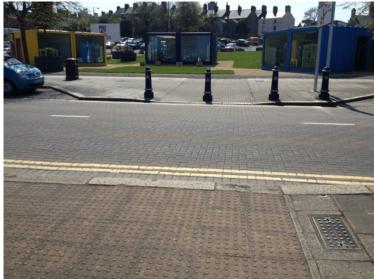
At the junction of Southwell Road/Greys Hill dropped kerbs have been provided. However these are not in-line and no tactile paving has been provided.
