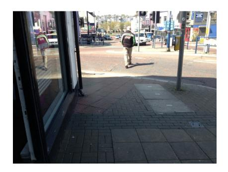
There is an in-line uncontrolled crossing at the junction with Mill Row. There is non-standard (over) use of tactile paving. There is significant damage to the tactile paving suggesting illegal or inappropriate pavement parking which potentially obstructs pavement width on occasions.
