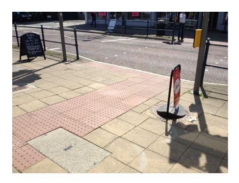
There is an in-line uncontrolled crossing at the junction with Beatrice Avenue. There is a lack of contrast between the tactile paving and the pavement surface. Also a variety of coloured tactile paving has been used.
