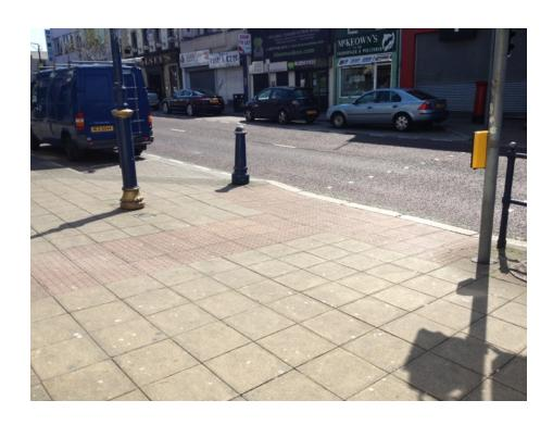
A-boards restrict access to what is a reasonable in-line uncontrolled crossing at the junction with Albert Street. The tactile paving does not however contrast with the surrounding pavement.
