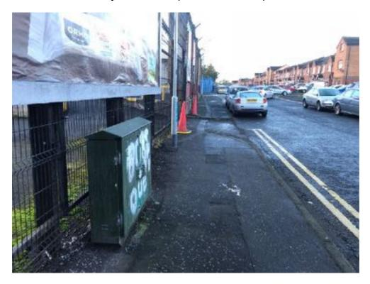
The condition of the northern section of footway is very poor and parked cars reduce its width.
