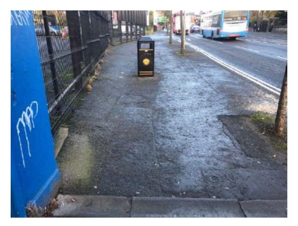
No tactile paving to warn pedestrians with a visual impairment has been provided at the vehicle exit to the garage on Clifton Street.
