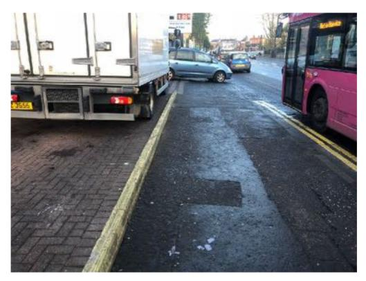
There is an in-line uncontrolled crossing at the junction with Trinity Street. Tactile paving has been poorly laid and lacks the appropriate depth and width particularly on the city centre side partly due to the radius of the kerb.
