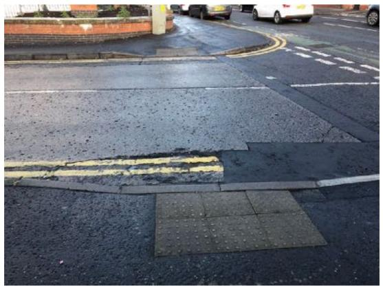
There is a gated vehicle entrance to facilities connected to the Mater Hospital. Although the kerb has been dropped, no tactile paving has been provided to alert pedestrians with a visual impairment.
