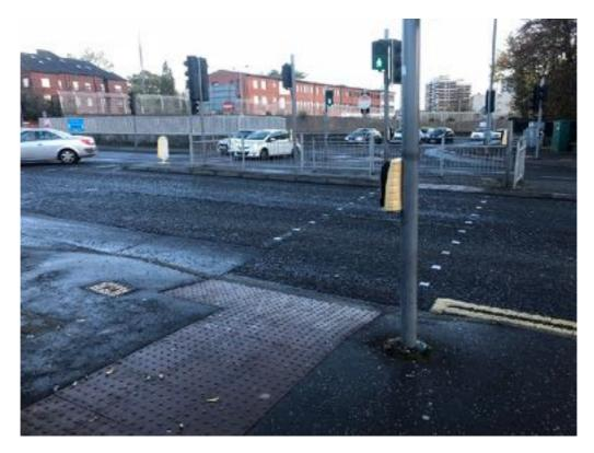
Although broad the footway on the eastern side between the eastbound onslip and Stanhope Street after this point is rough and uneven. A large dish drainage channel runs down its centre.
