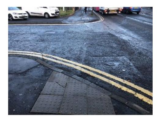
A bin has been placed in the centre of the eastern footway, creating an obvious hazard. A deep transverse dish drainage channel is also a hazard.
