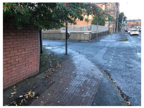
There is a staggered controlled crossing with traffic island across Clifton Street at this point. The incorrect positioning of the control boxes and the single tile depth of tactile paving on the island is problematic.
