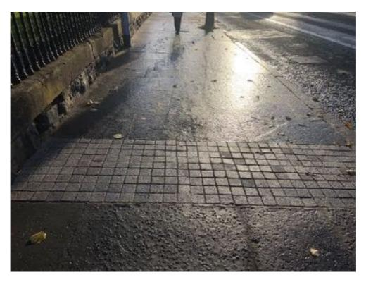
The design and placement of a cycle hoop creates a potential hazard. The main pedestrian entrance to the jail retains granite kerbing some of which represents a potential trip hazard.
