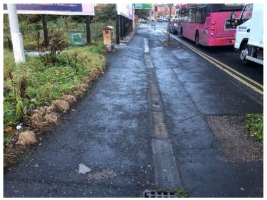
There is an in-line uncontrolled crossing across the junction with Stanhope Street. Tactile paving depth has been reduced in sections due the radius of the kerb at the junction.
