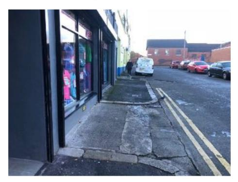
There is no footway on large parts of the northern section of Trinity Street because of the entrance to the garage with no tactile warning provided for pedestrians with a visual impairment. The section footway that is provided is obstructed by parked vehicles.
