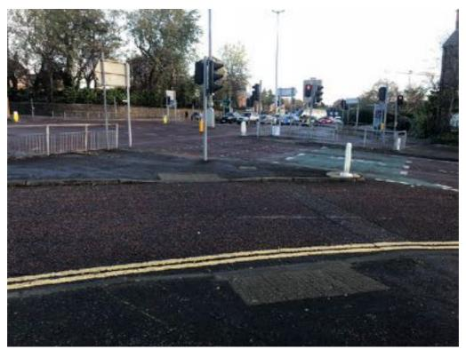
The tactile paving on the eastern footway does not contrast with the surrounding paving on the controlled crossing across Donegall Street on the eastern footway.
