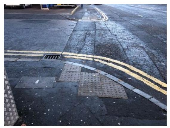
The footway approaching Carrick Hill is rough and uneven and includes dish drainage channels. There is a substantial section of dropped kerb to allow access to a garage.
