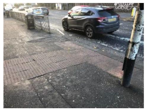
The Zebra crossing has a central refuge with tactile paving and the beacon located centrally, creating a hazard. The tactile paving on the western side has also been laid incorrectly.
