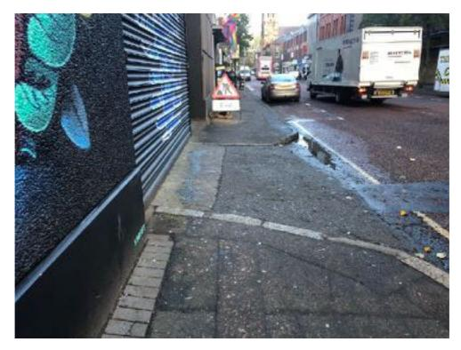
There is an uncontrolled crossing across the junction with Union Street. Whilst in-line and using the correct tactile paving the carriageway surface is in poor condition creating a potential hazard.
