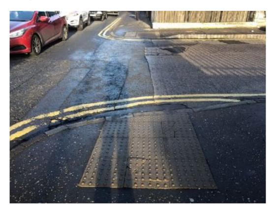
There is a Zebra crossing across Clifton Street close to Carlisle Circus. The tactile paving has been laid incorrectly on the eastern side and the footway condition is poor.
