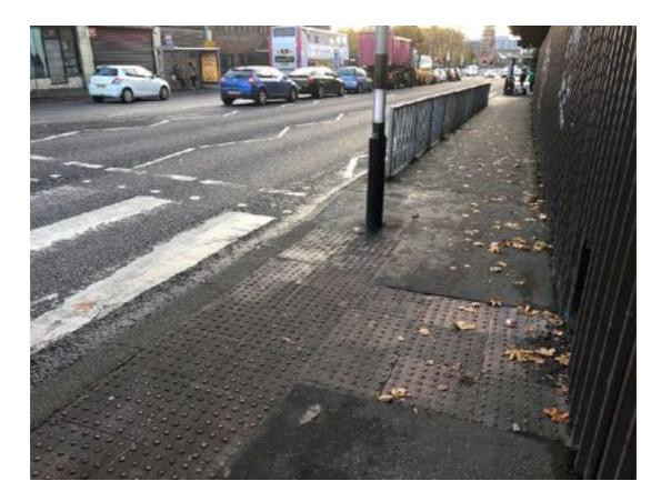
On the west side there is a controlled crossing across the exit from the Westlink onto Clifton Street. The control box at city centre side of the crossing is not beside the tactile paving.
