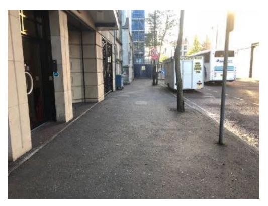
Ramped access to the temporary footway associated with the redevelopment of the University of Ulster has been provided. The design and condition of the ramp is poor and will be a hazard to some disabled people.
