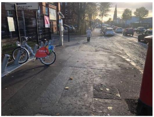
There are a number of other vehicle entrances across the footway at the front of the hospital. Each uses granite kerbing which is dropped but does not provide flush crossing. No tactile paving is provided at these crossings. Design and positioning of cycle hoops is problematic.
