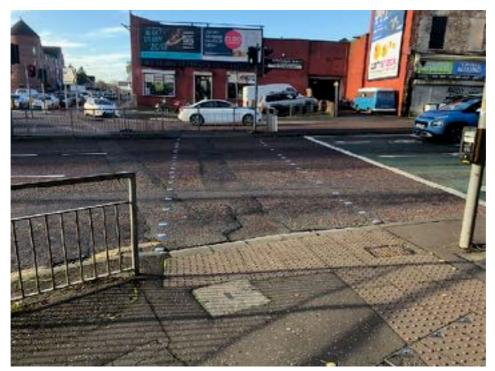
The footway surface on the eastern side of Clifton Street is rough and uneven and is narrowed below acceptable standards at points by the positioning of trees and street signs.
