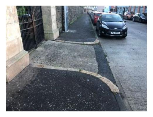
The southern section of footway is clutter free and is in much better condition. However there is a lengthy section of footway flush with the carriageway which could potentially allow someone with a visual impairment to stray onto the carriageway.
