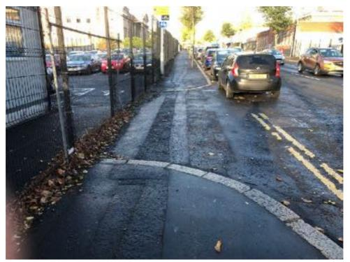
There is an in-line uncontrolled crossing across the junction with Florence Place. The depth of the tactile paving does not meet acceptable standards, partially due to the radius of the kerb. The carriageway surface is rough and uneven.
