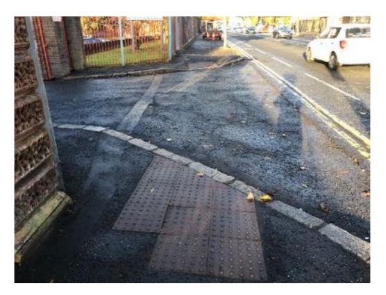
The footway on the western side approaching Agnes Street is rough and uneven. A temporary, large roadworks sign blocks the footway at this point making it difficult or impossible for many users to use the footway at the time of the audit.
