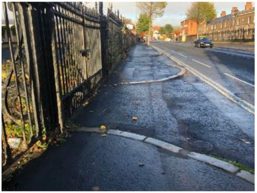
There is an uncontrolled crossing at the entrance to the Crumlin Road Health Centre. The tactile paving is the wrong colour and is not correctly aligned.
