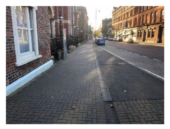
There is an uncontrolled crossing at the junction with Donegall Lane. The tactile paving on the does not meet design requirements in terms of depth. There is a significant section of this junction where the kerb is flush with the carriageway without tactile paving.
