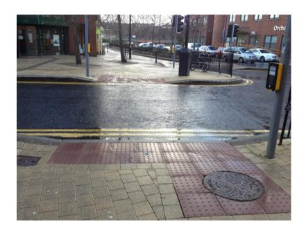
At the junction of Foyle Street and Water Street there is controlled crossing. As with 5 above the tactile tail should extend to the building line. Also there is an associated traffic island which includes non-standard use of tactile paving.
