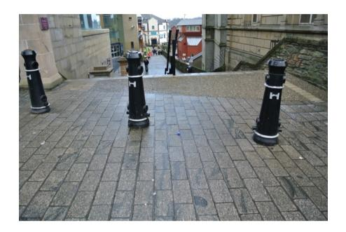
There is a reasonable in-line uncontrolled crossing at the junction of Market Street and Newmarket Street. The tactile paving is non-standard and fails to provide adequate contrast.
