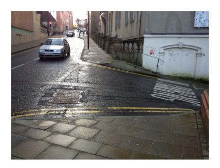
There is a controlled crossing near to the entrance of Foyleside Shopping Centre. The control button on the crossing is too far from the tactile paving. Bollards in the vicinity have no contrasting band.
