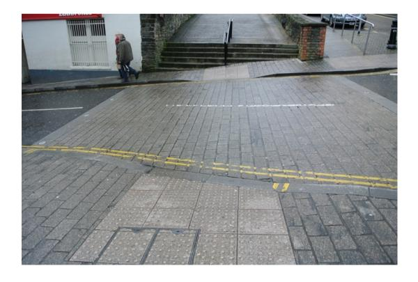
There is no corduroy hazard paving around the steps in this area. Some attempt has been made to include a white band on bollards but this is not wide enough to provide an acceptable contrasting band.
