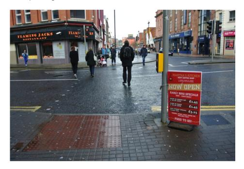
At the same junction there is a controlled crossing over Strand Road. Once again there is non-standard use of tactile paving and the control box is too far from the paving.
