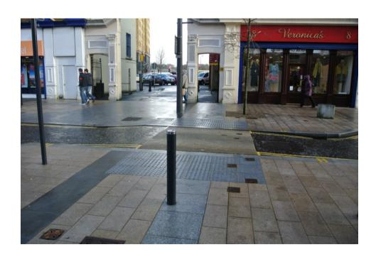
There is an in-line uncontrolled crossing at the junction with Sackville Street. Two different colours of tactile paving are used on one side, non-standard paving on the other. Bollards on one side present an additional obstruction.
