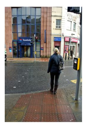
At the same junction there is controlled crossing at the eastern junction with Great James Street. Once again there is non-standard use of tactile paving and the control box is too far from the paving.
