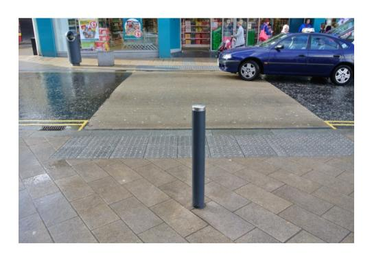
The use of dish drainage channels to demark the pedestrian and road surfaces in areas of Waterloo Place is not ideal but is preferable to no delineation.
