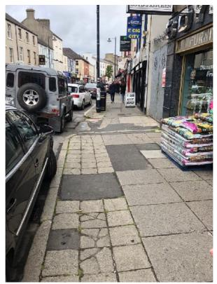
The footways here are in poor condition and include older concrete dish drainage channels.
