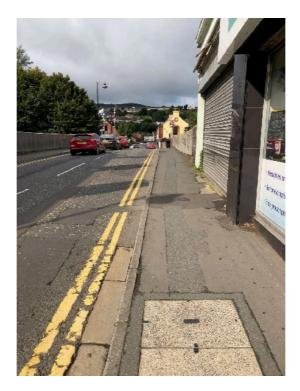
Drop kerbs have been provided without tactile paving at the entrance/exit to the car park and bus centre. These are not in line and there is no pedestrian phase provided at the traffic lights.
