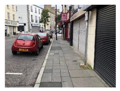
The footway on the western side of Hill Street is relatively narrow and in a poor condition. Concrete dish drainage channels have again been used.
