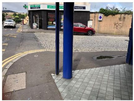
No tactile paving has been provide across St Mary's Street at its junction with Mill Street.
