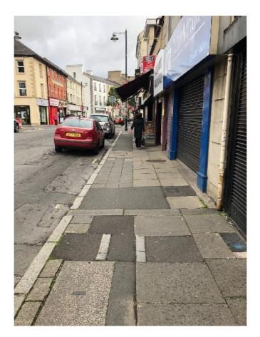
No tactile paving has been provided at the junction with Mill Street on the eastern side of Hill Street. The location of street furniture creates potential hazards and could be improved.
