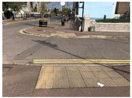
There is a further uncontrolled crossing with appropriate tactile paving across John Mitchell Place beside the First Presbyterian church. The footway is broad at this section on the eastern side , however street furniture including bins could be positioned better.
