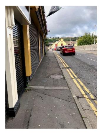
At the signalised junction with the car park on the southern footway, dropped kerbs have been provided with no tactile paving. A pedestrian phase has not been provided with the traffic lights.
