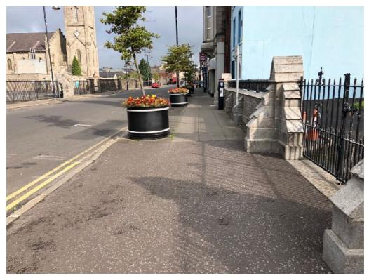
The footway along this eastern section is in poor condition with old dish drainage channels. A-Boards create additional obstacles.
