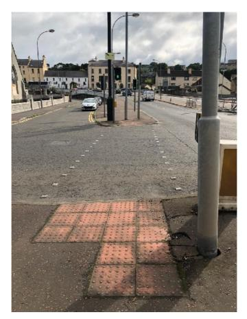
An uncontrolled crossing is provided to cross the side street close to the junction with William Street on the eastern side of John Mitchell Place. Appropriate tactile paving has been provided.
