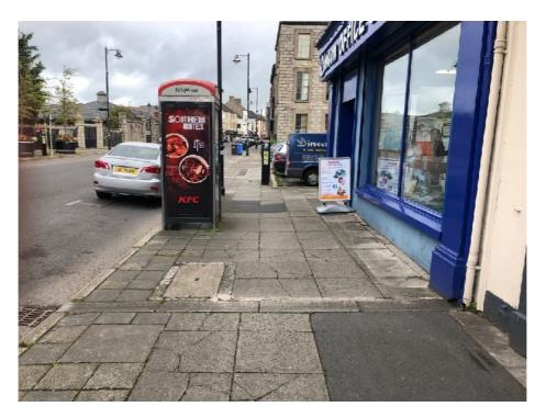
There is no tactile paving at the junction between John Mitchell Place and St Colman's Park. Cars parked on St Colman's Park overhang the footway creating a potential hazard.
