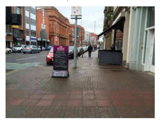
The pavement in this area is generally wide, however the surfaces in places are uneven and dish drainage channels are used.
