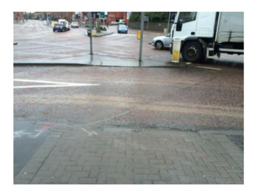
There is a controlled crossing across North Queen Street at this junction which is reasonable. However as with paragraph 48 the inclusion of an uncontrolled crossing creates a challenge. The non provision of tactile paving is not satisfactory.
