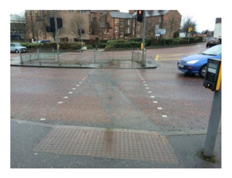
The uncontrolled crossing at Frederick Street at this location has no tactile paving on one side of the crossing.
