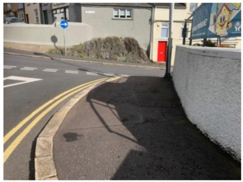
Tactile paving is completely absent at all uncontrolled crossings in the areas of the proposed public realm, even where the kerb has been dropped.
