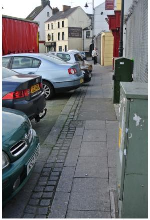
70 There is a non-standard in-line controlled crossing at the junction of Merchants Quay and Sugar Island. The tactile paving on the northern side of the road do not appear to lead to the end of the pavement which is narrower than the tactile. This is confusing and potentially hazardous for people with a visual impairment.
