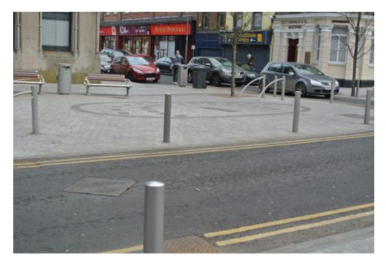
28 The flush surface between pavement and road continues for a short distance along Hill Street. Unmarked bollards and a dish drainage channel provide a less than satisfactory delineation.
