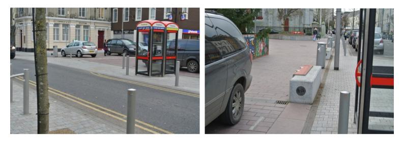
26 As with Margaret Square in-line uncontrolled crossings have been provided. Once again pedestrian accessibility could be improved by extending the length of the tactile paving over the width of the crossing.
