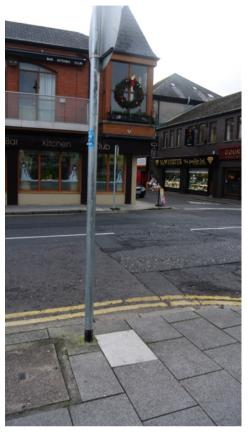
8 At the junction of the bridge linking Kildare Street with Monaghan Street dropped kerbs have been provided. These are not inline and have no tactile paving. The dropped kerbs direct people into the middle of a very busy junction and therefore represent a hazard.
