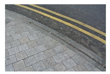
21 There are four in-line controlled crossings on the square. These follow good practice in relation to the provision of this type of crossing. However given the "shared" nature of the area consideration should be given to extending the length of the tactile paving at these crossings.
