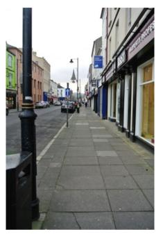
20 A recent public realm scheme has improved surfaces around Margaret Square. The square is busy with parking for taxis and cars. There are no kerbs in the area with dish drainage channels used to delineate between the flush road and pedestrian surfaces. This type of delineation is not something Imtac would recommend.
