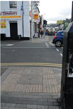
59 There is a reasonable example of a controlled pedestrian crossing just after the Kilmorey Street junction. Whilst the paving a has been renewed and correctly installed the signals have not and have no tactile rotating cones.
