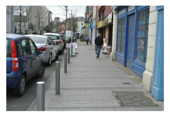
29 Approaching the cathedral on Hill Street the public realm scheme ends. At this point there is an inline flush uncontrolled crossing. The use of tactile paving at this crossing is incorrect and there is no contrast between the tactile and surrounding paving. A kerb is reintroduced after this crossing.
