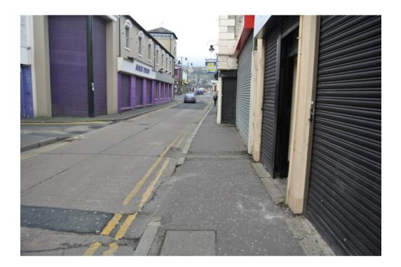
38 The absence of dropped kerbs means there is no accessible opportunity to cross Mill Street at the junction with Georges Lane. The pavement surfaces are poorly maintained.
