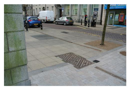
30 There is another inline flush uncontrolled crossing at the entrance to the Cathedral. The use of tactile paving at this crossing is incorrect and there is no contrast between the tactile and surrounding paving. The paving in this area is in a poor state of repair.
