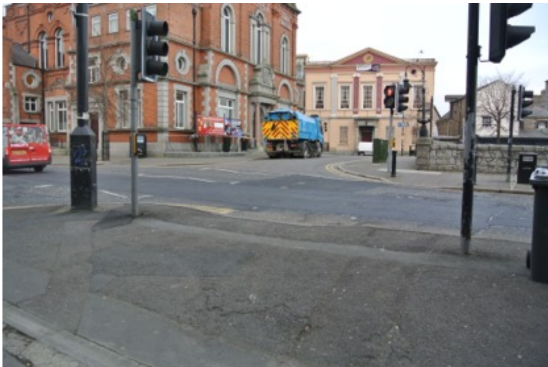
Picture 3: An example of old infrastructure, a controlled crossing in the heart of Newry City Centre without even basic tactile paving
