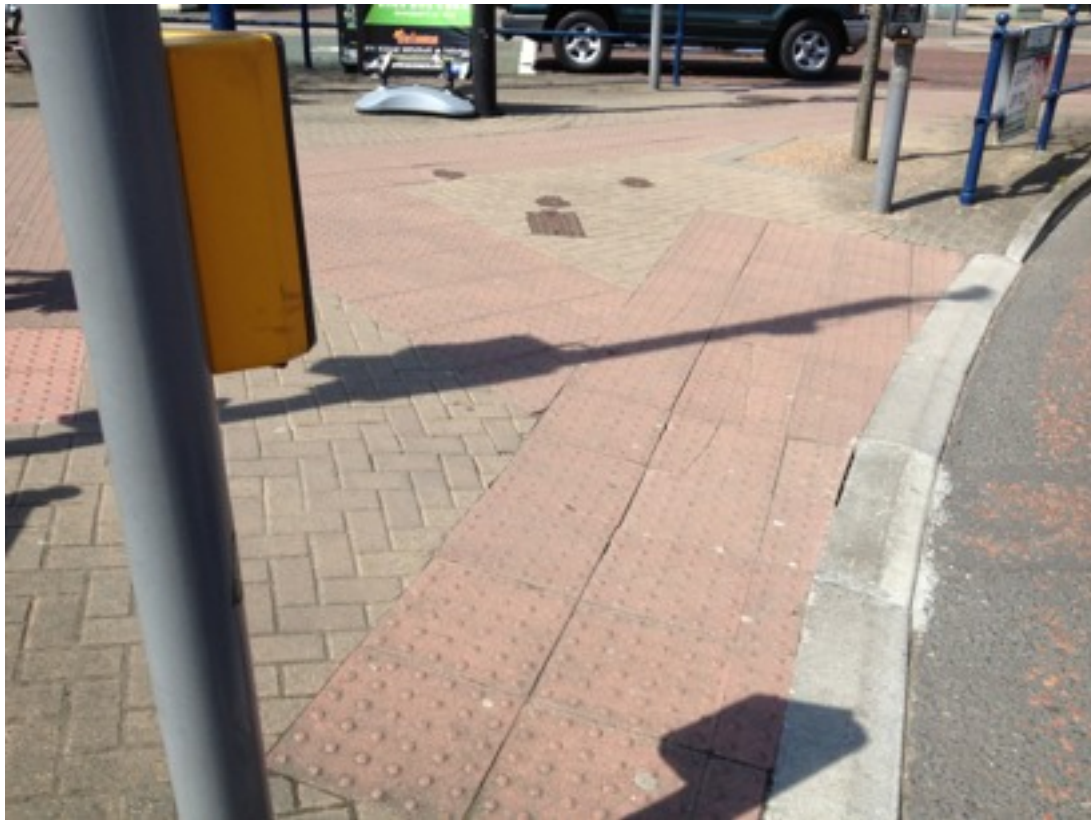
Picture 4: Incorrect use of tactile paving at a busy traffic island in Bangor creates a confusing and potentially dangerous junction for people with a visual impairment.
