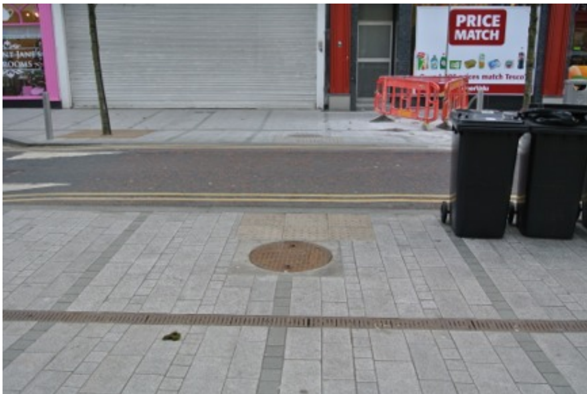
Picture 7: The benefits of wide, raised crossings in Newry city centre are lessened by clutter and the limited use of tactile paving.
